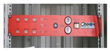
Representing the future in cabinet protection; Inrack fire suppression system is a self contained automatic fire extinguishing system for rack enclosures and equipment cabinets, which can be used in all industry sectors to protect valuable assets and critical systems and processes.
