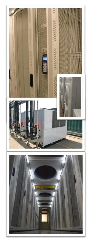
(#1) 8 x WIRC units @ 500w = 4kw, 3kw of water pumps and 5kw of free cooler fan energy = 212kw total for 200kw of sensible cooling – (free cooling metric based on Southampton UK Winter period).
